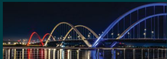
Frederick Douglass Memorial Bridge , Washington, D.C., U.S. Design Build EOR for SCB (Archer Western & Granite Construction)
